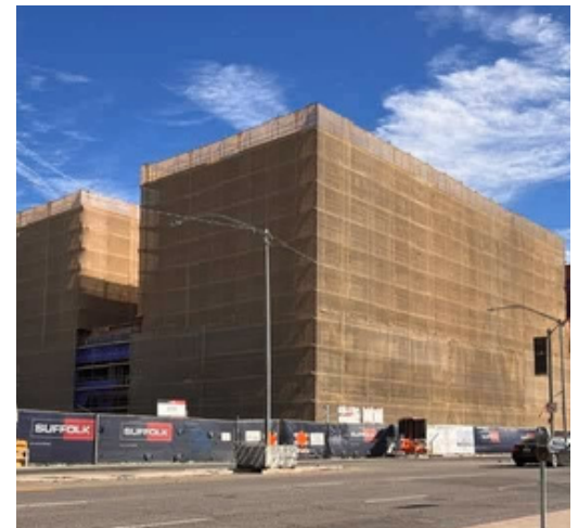
CRCD's Evermont housing development under construction
